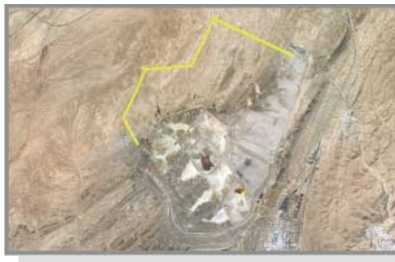
Figure 4. The current tailings dam and its proposed extension if mining operations continue to 2016.
