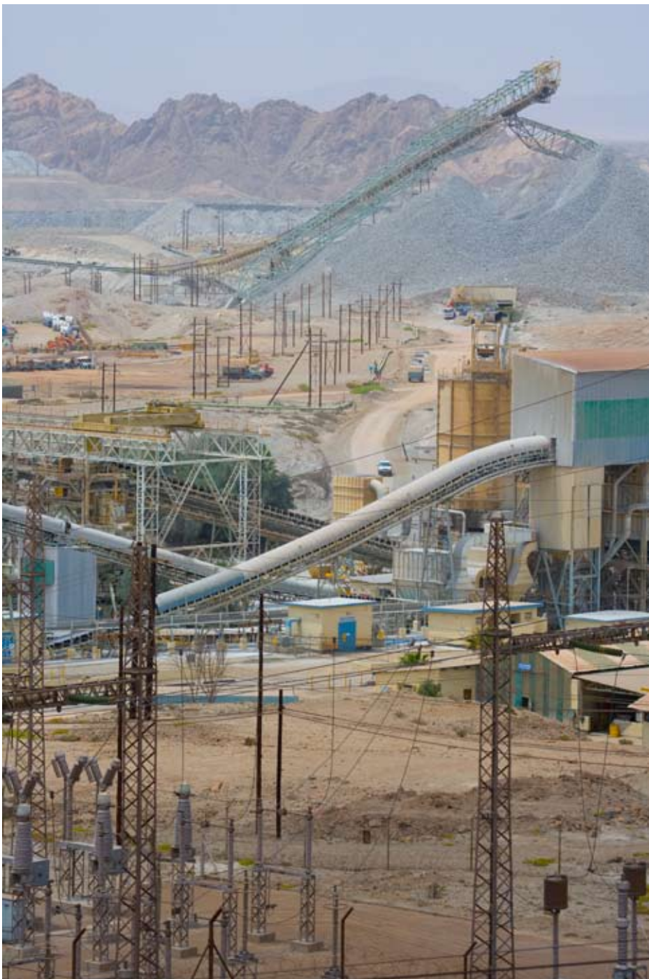
Mining activity at Rössing with a view of the coarse ore stockpile and the fine crushing plant.
