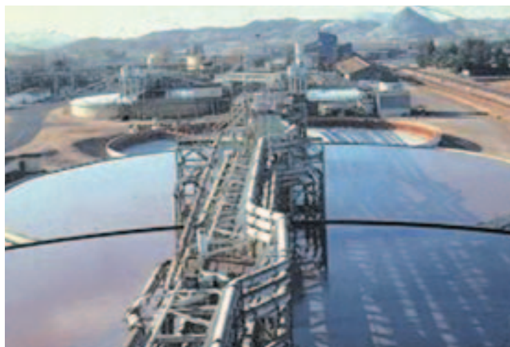
The thickeners or Counter Current Decantation tanks. Photo courtesy of Rössing Uranium
