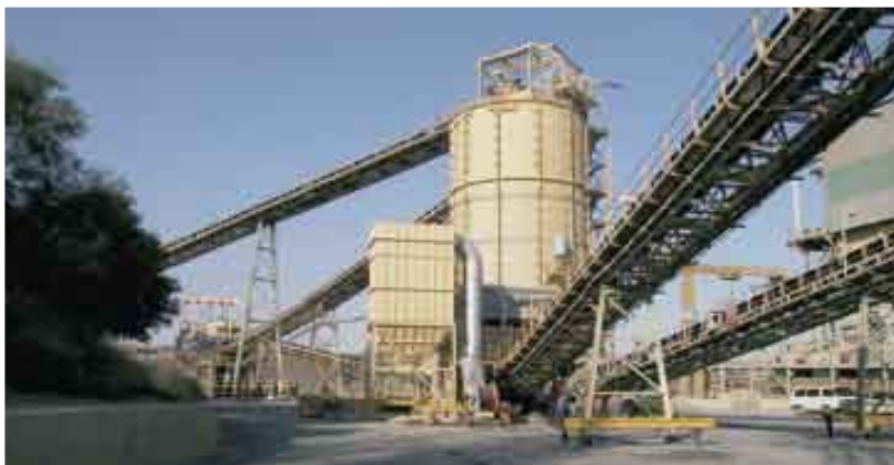
DUST: A new dust collector was installed at the pre-screening plant and is one of many control points to monitor dust on site.
