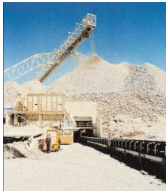
The coarse ore stockpile, which has a live capacity of 80 000 tonnes and a total capacity of 400 000 tonnes. Coarse ore is withdrawn from the stockpile by seven vibrating pan feeders feeding directly to a coarse ore reclaim conveyor.
