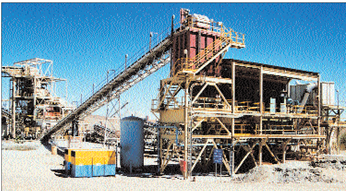
The pilot ore sorting plant with (in left background) the pre-screening plant.
